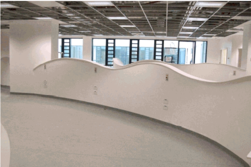
Maternity & Oncology Unit, North Staffordshire Hospital (During Construction)
